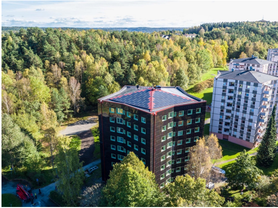
Figure 1: Kollektivhuset Stacken with BIPV façade and roof next to neighboring unrenovated “star” buildings. Photo courtesy of Badenfelt and RISE.
